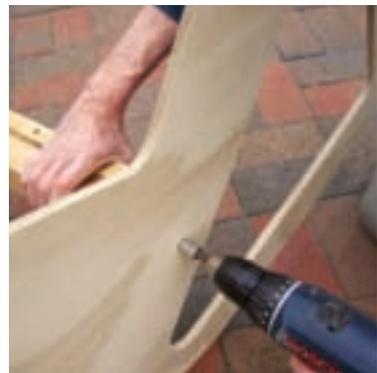
**3c. IMPORTANT:** With the seat and back pieces flush with the wide side of all 3 cross braces, fasten the back to cross brace A with three #8×1½" flathead wood screws. These screws prevent braces A and B from rotating; your weight will keep brace C fixed.
